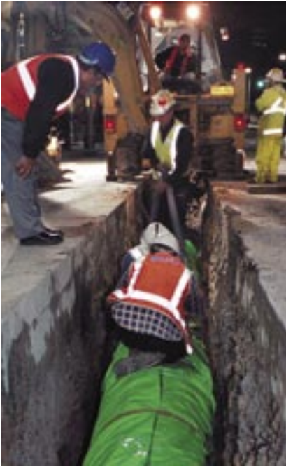
Replacing a section of water main to help with leakage reduction
