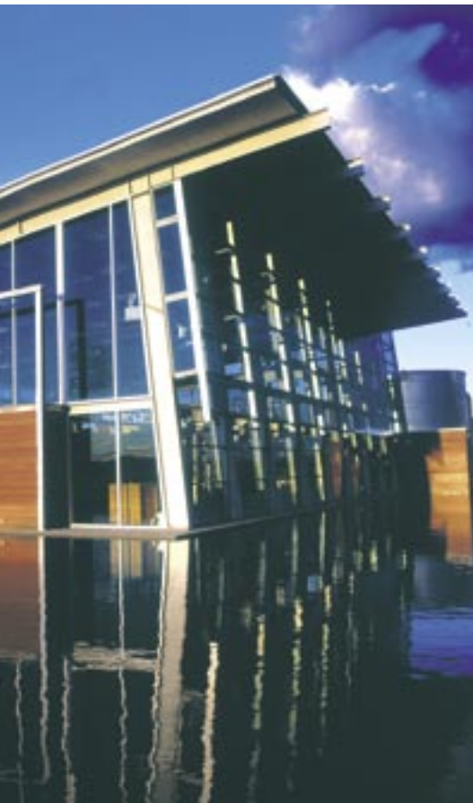
The recycled water treatment plant at Sydney Olympic Park, used to treat sewage and stormwater for reuse for irrigation and toilet flushing
