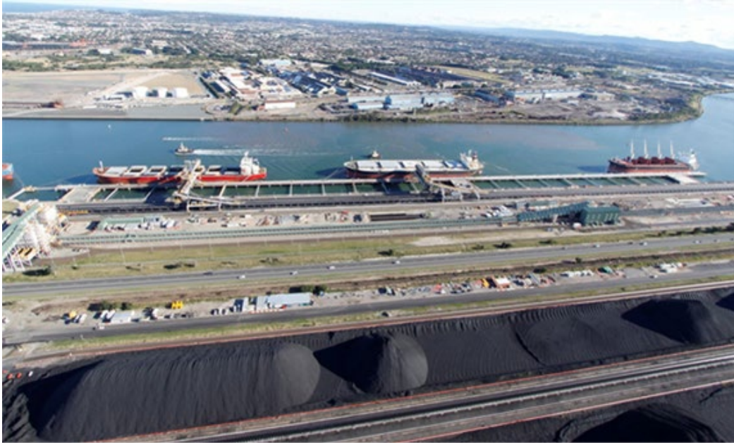
Figure 4: Shiploaders and berths at NCIG Terminal
