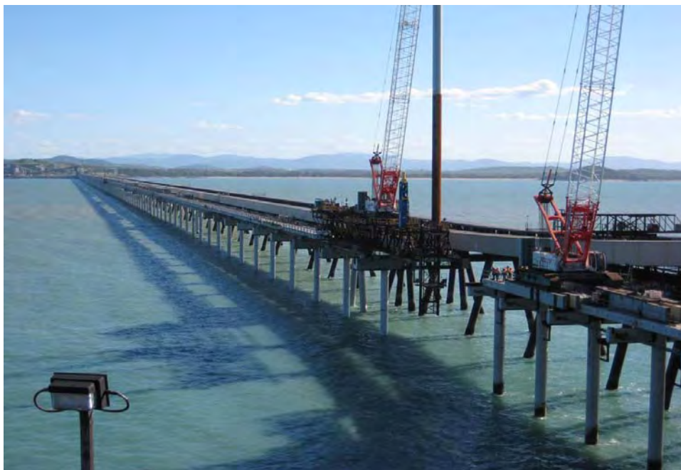
The last pile driven on the jetty triplication, 7X Project – DBCTM 2009
