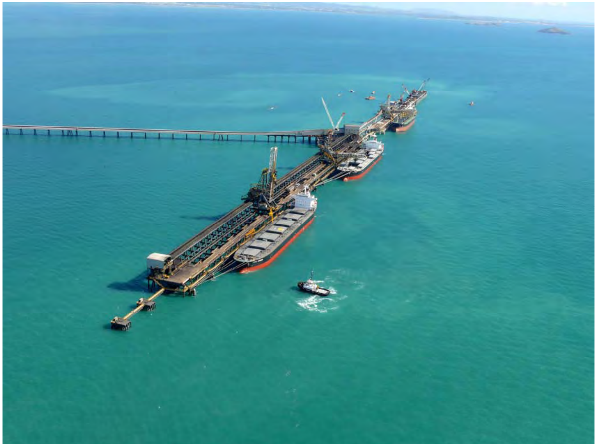
DBCT 4 Berth outloading configuration – DBCTM 2008
