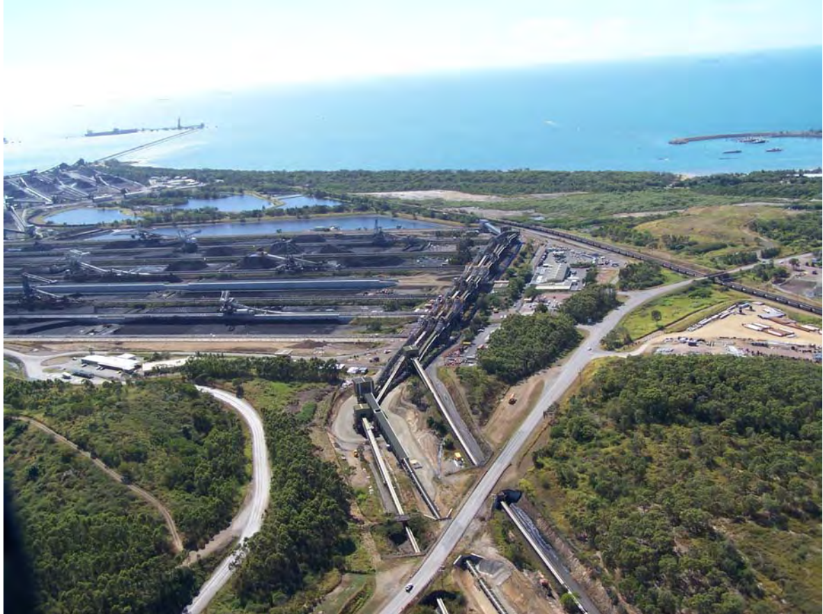
DBCT inloading galleries and stockyard
